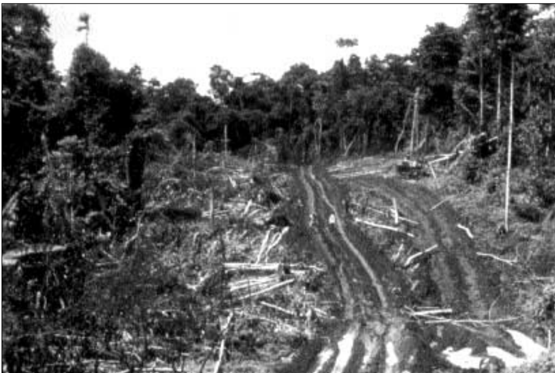
Road construction, Ecuador
