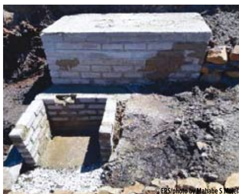
Above - A formal collection chamber sits behind the access point where water can be collected from the tap.
