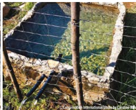
Above - This collection chamber receives water from the pipes at the back of the tank and the overflow at the front is available for collection as needed.
