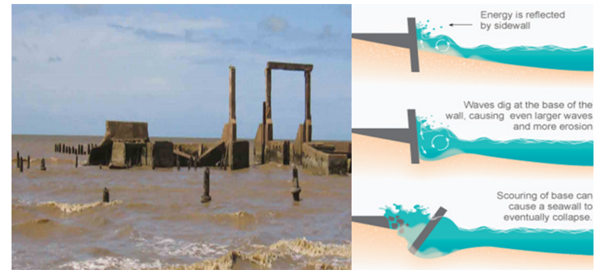
Figure 5. Failure of hardened sea defence structure in Guyana (source: Winterwerp et al. 2013 (left); USACE 2019 (right))
